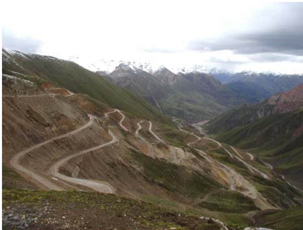
Picture 3: Strategic road-building to improve access and reduce isolation
